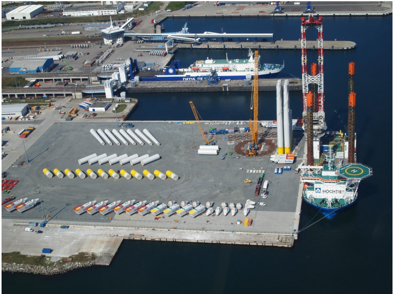
Figure 7: Onsite port storage for wind turbine components [23]
