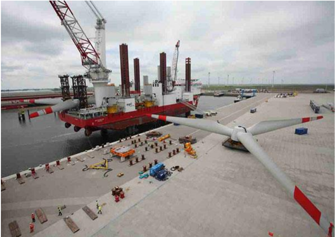
Figure 17: Hub with blades in star configuration assembled at the port for the Borkum West II Windfarm, Germany [80]
