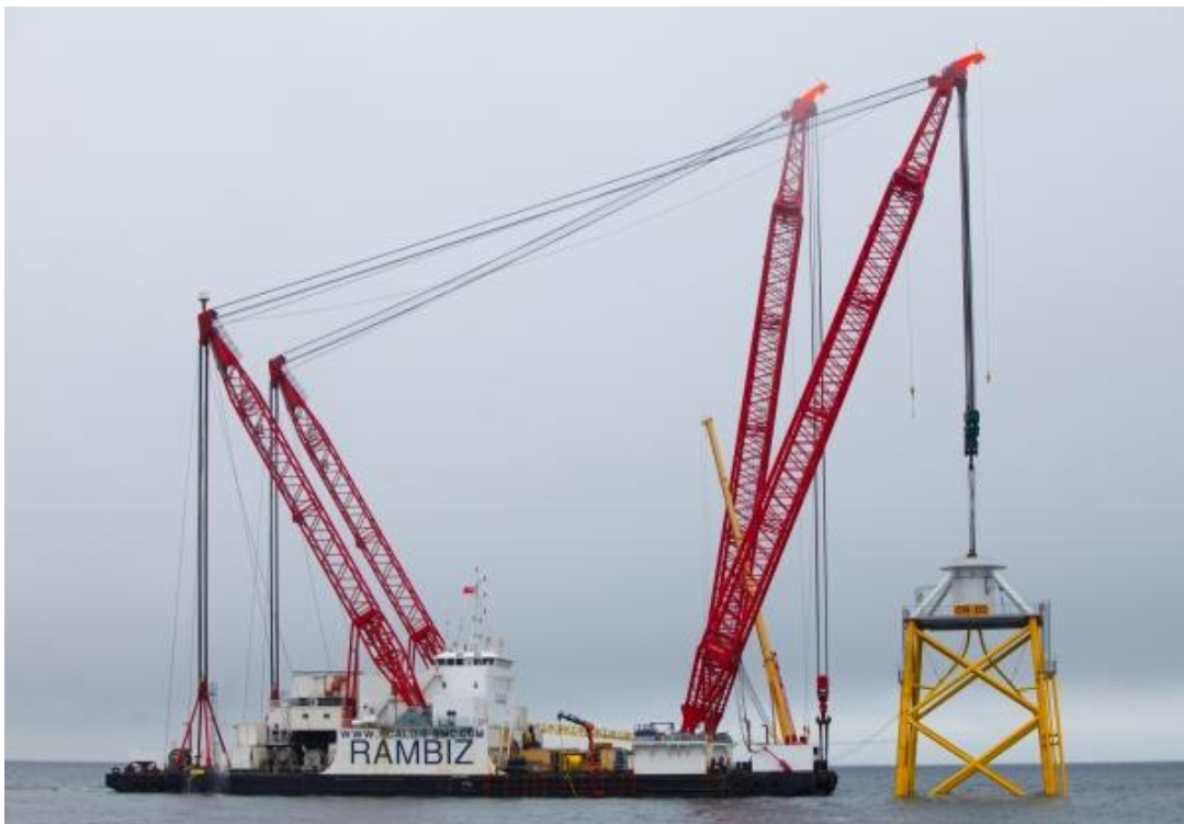
Figure 20: Scaldis Salvage & Marine Contractor's heavy lift vessel Rambiz was used to install the jacket foundations for the Ormonde project located at the North West coast of the UK. Image courtesy of Vattenfall [41]
