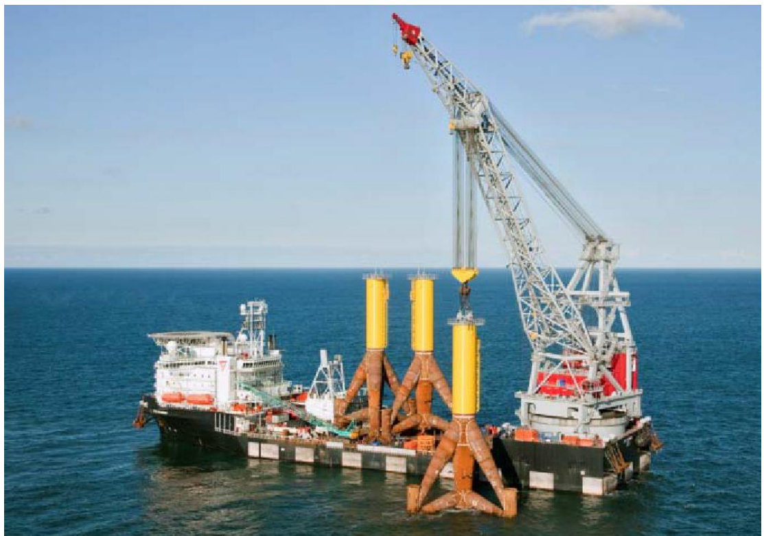
Figure 22: 5000 tonnes mono-hull DP crane vessel Oleg Strahnov, installing wind turbine foundation tripods at Borkum West II Windfarm, Germany [43]
