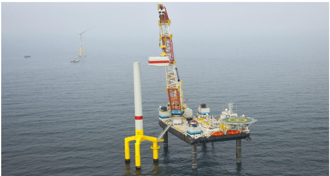
Figure 18: JB-117 installing the nacelle [37]
