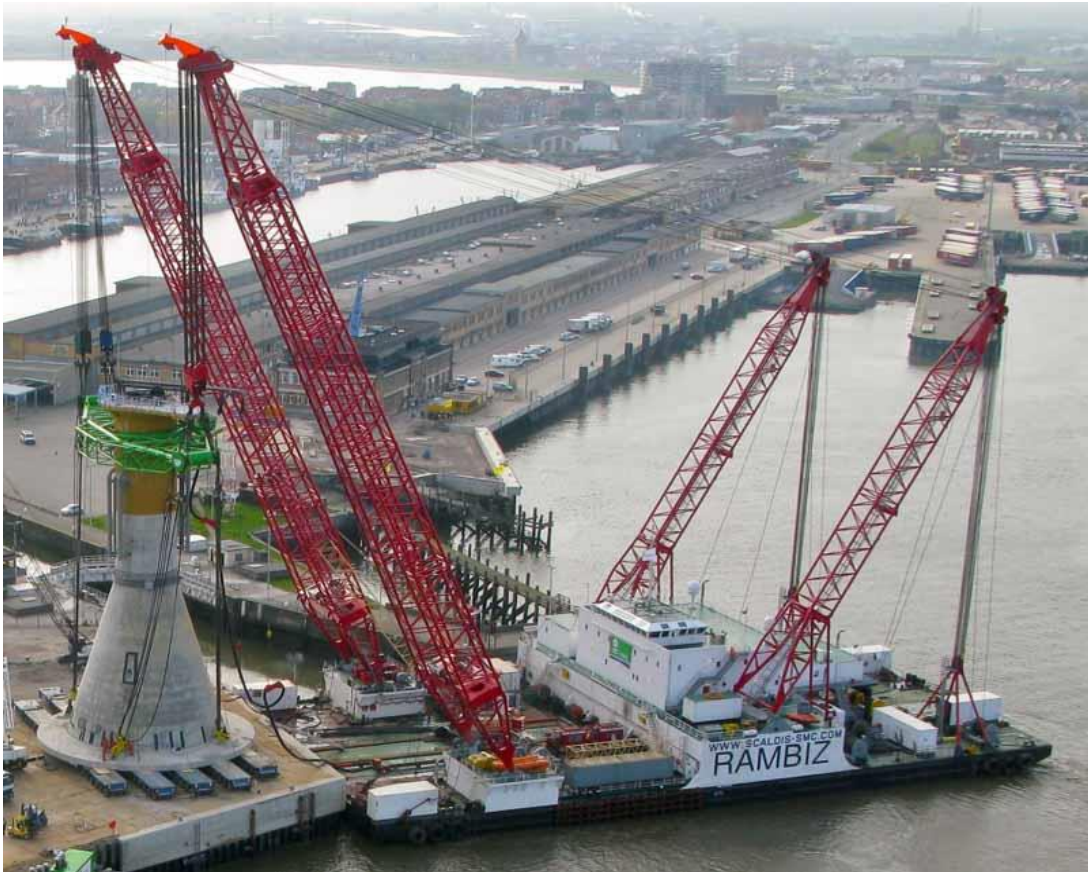
Figure 19: Rambiz lifting GBF at port of Oostende [40]
